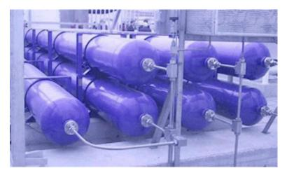
Storage vessels for Hydrogen, Design pressure: 450barg
